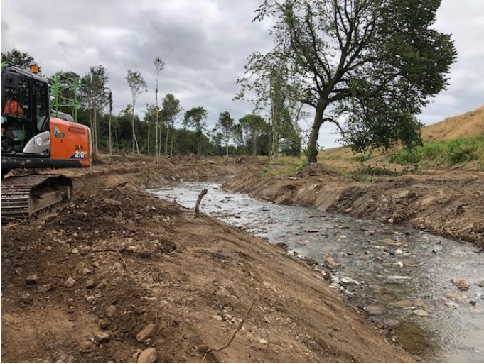
General View of works. (Jim Kerr)
