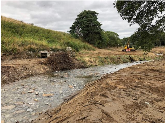
Bronie Scottiesly Weir removed. (Jim Kerr) (Note the location of the old lade take-off on the left centre of the picture.)
