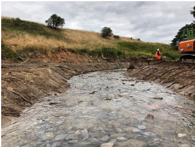
General View of Works. (Jim Kerr)
